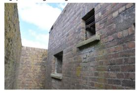
Original iron grilles are corroded and mostly missing.
