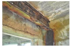
Beam is heavily corroded and causing damage Replace beam to tower to building
