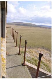
Existing handrail is badly corroded
