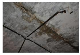
Existing roof slabs have various cracks and suffer from localised spalling of concrete cover to reinforcement.
