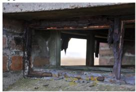
Original steel windows are largely missing and the few remaining ones are corroded beyond repair.
