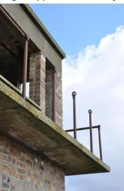
Existing balcony is in only fair condition and suffers from cracking (Structural Engineer's Report: 3.4.8)
