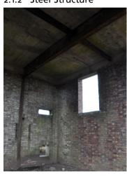
Existing steel frame has surface rust.
