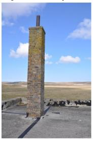
Structural Engineer's Report identifies possible issues with slenderness of chimney and proposes bracing of chimney.
