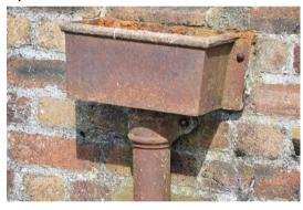
Existing cast iron hopper heads and downpipes in rusted condition or missing.
