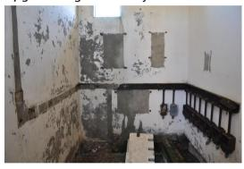
The existing electrical system has largely been stripped out. Some sections of conduit and original switchgear remain. In particular, some of the original runway lighting switchgear at first floor level.
