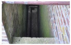
Existing roof drainage falls to channel in basement area with drain at NE corner.
