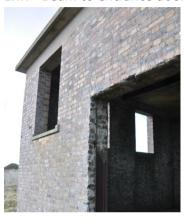
Entrance has been enlarged by removing beam and areas of brickwork to each side. NO STRUCTURAL SUPPORT HAS BEEN PROVIDED TO THE WALL ABOVE.
