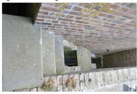
Stair has a number of broken treads and is too narrow to provide adequate access.
